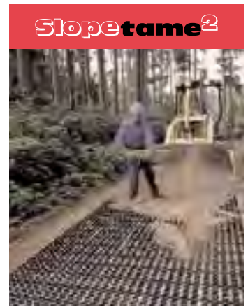
Slopetame 2 —much more than an erosion control blanket or mat—a completely integrated system of rings, grid, fabric, anchors, and vegetation to control erosion on some of the toughest slopes, channels, swales and more.
