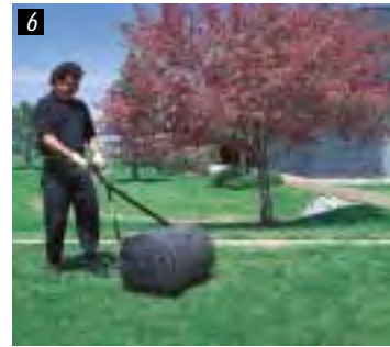
6 Roll sod with heavy roller.
