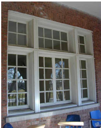
detail of facade showing current condition of windows
