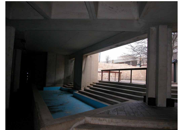
above: Plaza, lower level with fountain
