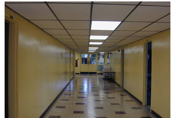
below: first floor corridor, North Building
