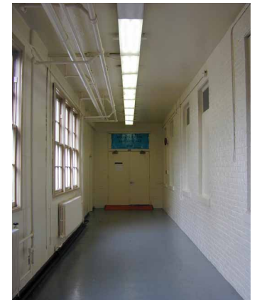
below: rear corridor of V Building
