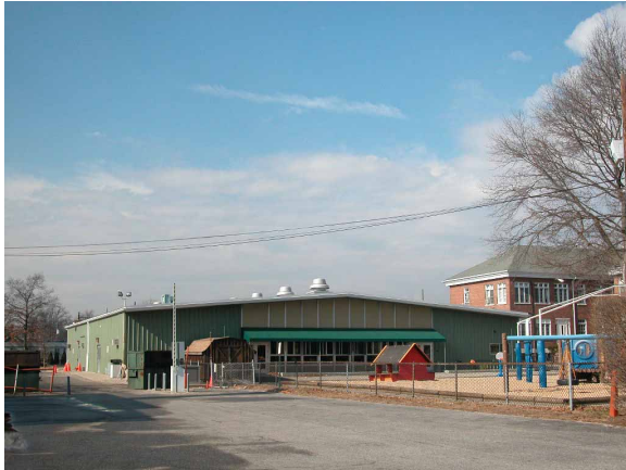
above: the Day Care Building (Greenhouse)
