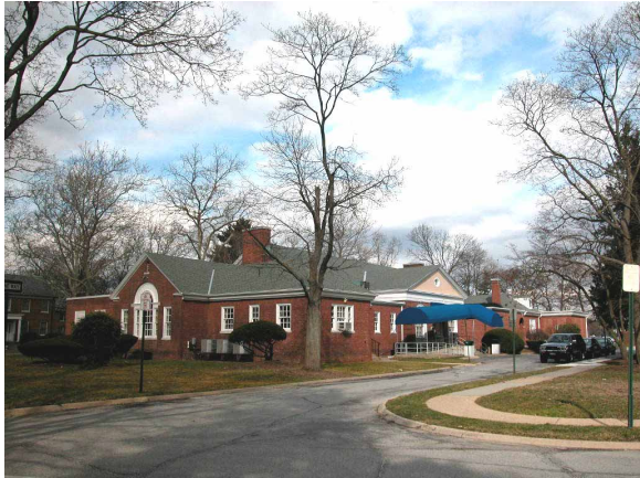
above: K Building, K Building, rear from East Road
