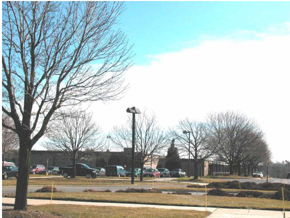
below: Physical Plant exterior from southwest
