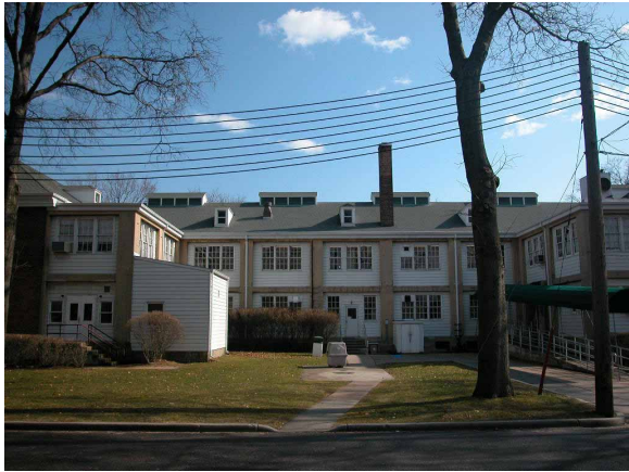
above: rear of V Building
