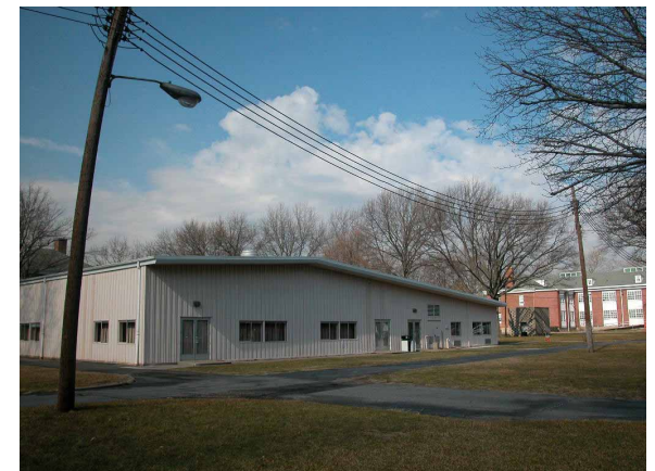
below: Q Building
