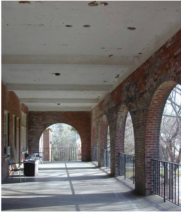
west loggia, Bradley Hall
