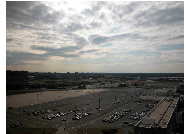
above: West Parking Lots 4A and 4B
