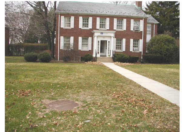
above: Manholes and overhead cables at Building 357
