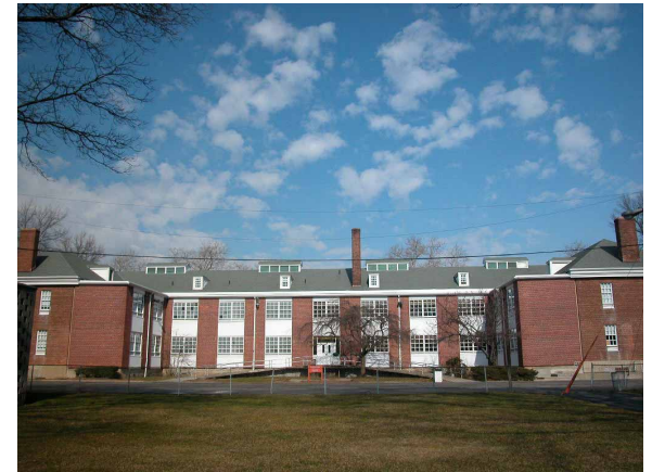
above: south facade, North Building
