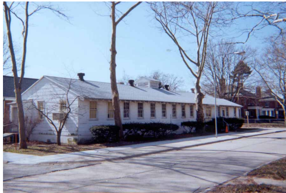
above: Building T-154 (Audio/Visual) from the northwest
