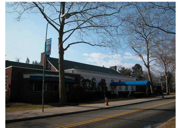
below: K Building, from Miller Avenue
