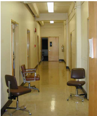
below: second floor corridor in V Building
