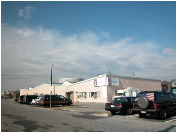
below: W Building from the southeast
