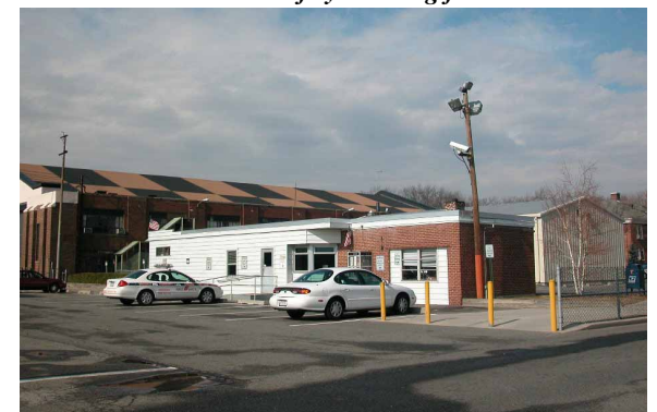
below: the Public Safety Building from the southeast
