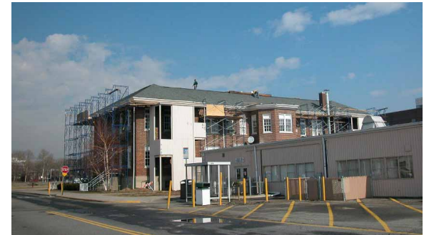
above: Student Union Building, rear
