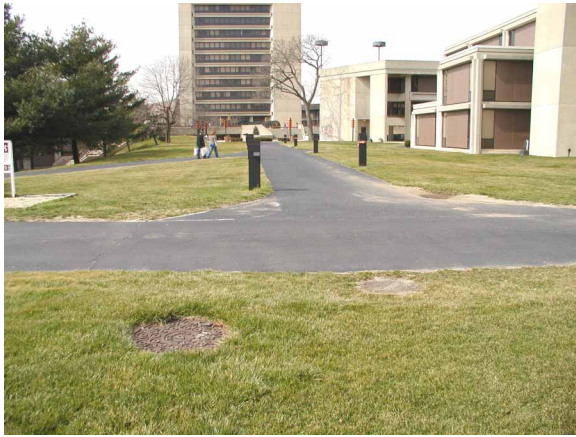
above: Utility manholes between Cluster Buildings
