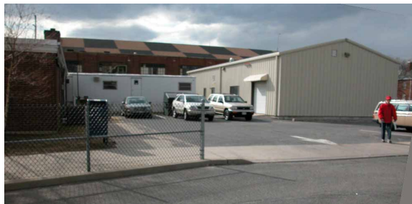
below: the Carpentry Shop in front of Z Building
